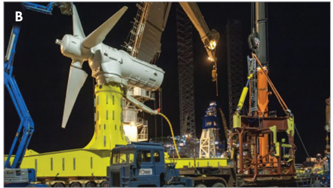
Figure 5: Horizontal-axis turbine. (A) Configuration of a horizontal-axis turbine. (B) One of the MeyGen Power Plant horizontal-axis turbines before loading on the ship for installation in the Pentland Firth (Scotland, UK). (Deign 2020)
