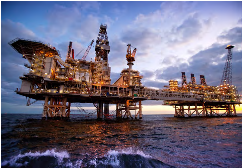
Picture 1: The Deep water Gunashli platform, offshore Azerbaijan.
