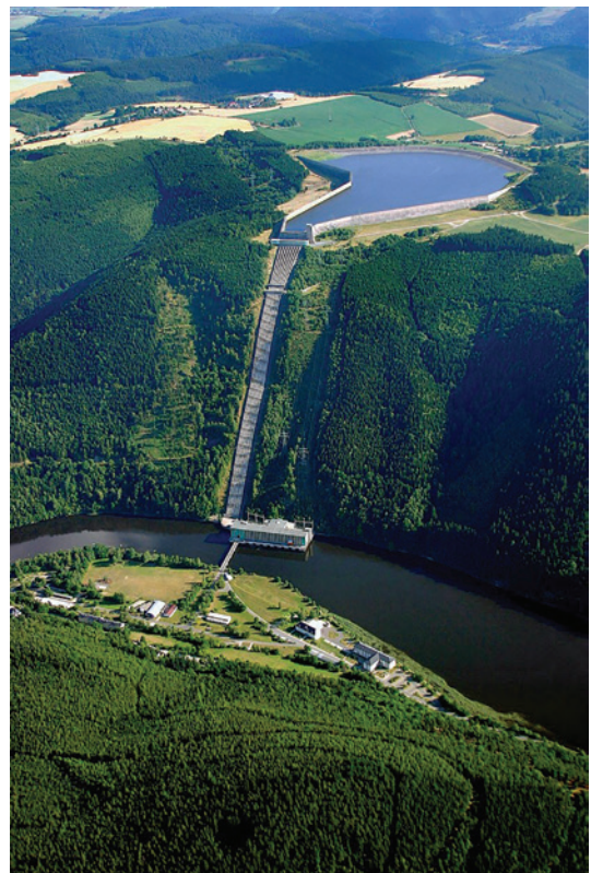
Figure 6: Pumped storage hydropower station "Hohenwarte II" in Thuringia, Germany which is owned by the Swedish company Vattenfall GmbH. The upper reservoir is filled with pumped water from the lower reservoir and river power plant during times of surplus electricity production. The water from the upper reservoir powers on demand the eight turbines in the machine hall, the height of drop is 304 meter (Flicker 2020; Vattenfall 2020).
