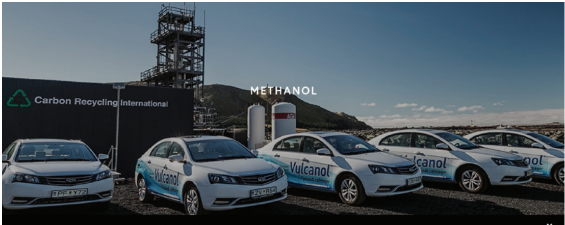
Figure 5: View of the Carbon Recycling International (CRI) plant in Iceland. Electricity is generated from geothermal sources and the carbon dioxide is captured from geothermal sources as well. Both raw materials are synthesized into methanol, which can be used as fuel (brand name "Vulcanol") in internal combustion engines in fuel cells and as chemical base material (Carbon Recycling International 2020).
