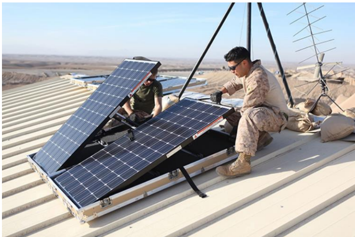
Figure 15: U.S. Marine Corps troops installing solar panels on a combat outpost in Afghanistan (November 2012) to provide power to radios, laptops and computers (Curwood 2017).
