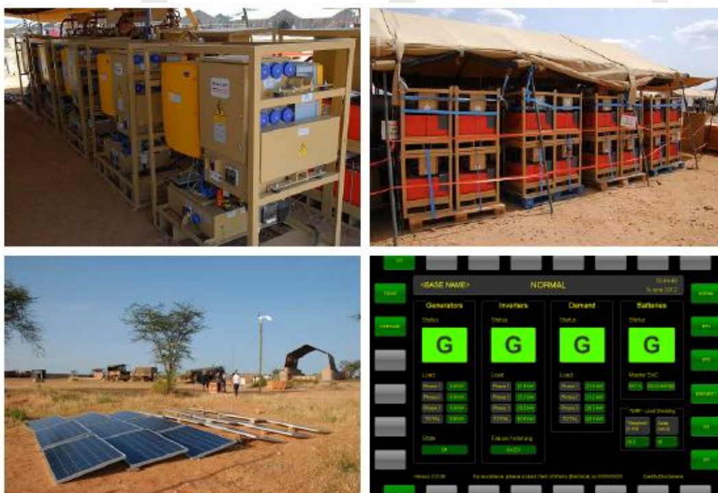
Figure 2 - Five Microgrid Modules in rugged frames fitted with plug and play connectors (top left), Batteries, also mounted in rugged frames with plug and play connectors (top right), a 4kW solar array with small wind turbine in the background (bottom left), main screen of the Deployed Energy Management System (DEMS) user interface (bottom right)
