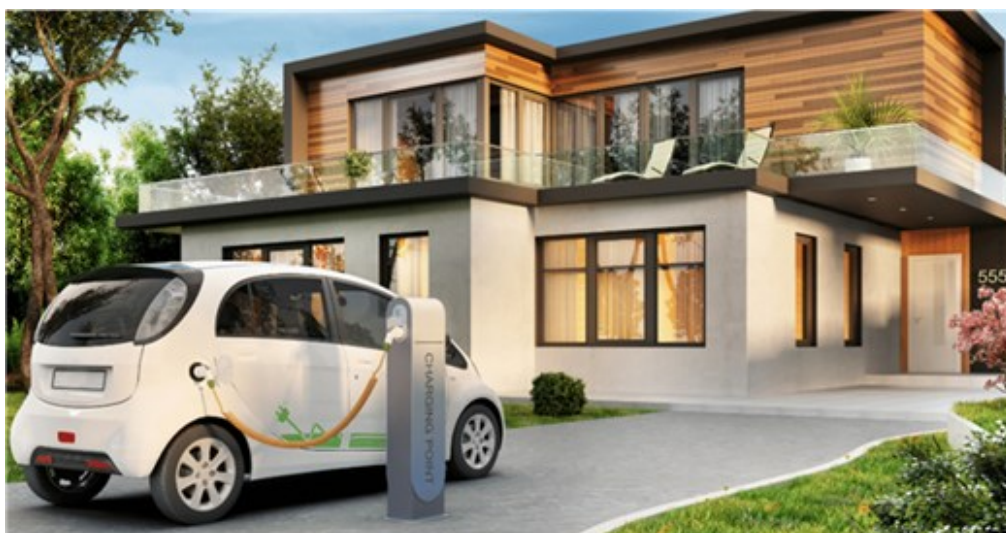
Figure 5. Repurposing used EV batteries for grid energy storage
