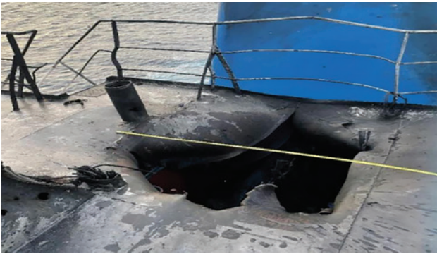
Figure 10. Damage Caused by a Drone Attack on the Oil Tanker (Mercer Street)
