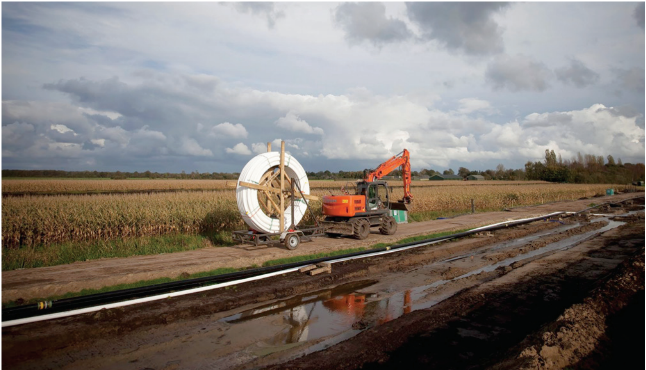
Figure 5: Flexible pipeline systems for hydrogen transportation and distribution by SoluForce (The Netherlands) 26 .
